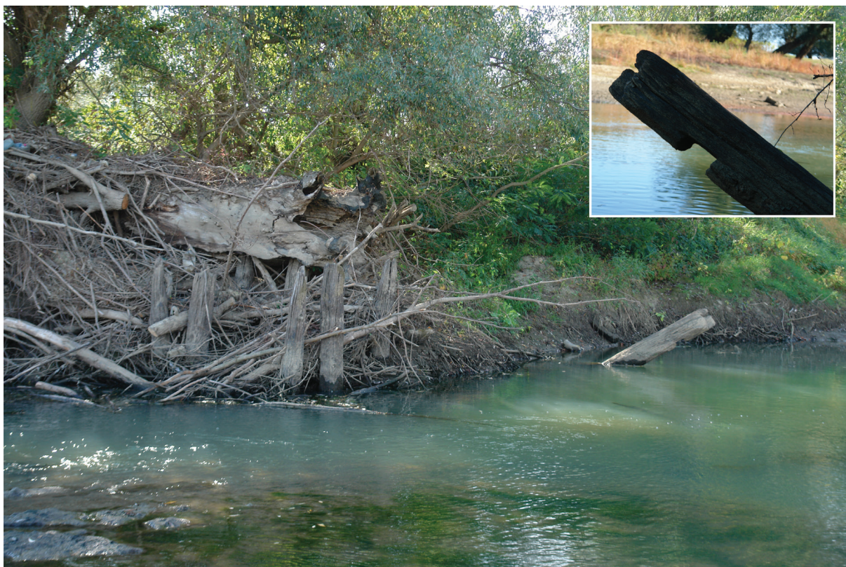
Fig. 34. Uliuc-Timiș 4B, riverbed view, eastwards (October 2019).
