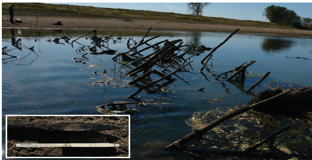
Fig. 26. Uliuc- Timiș 1, pole alignment forming the dam and the pole sharpening type (frame). Riverbed side photo (October 2019).
