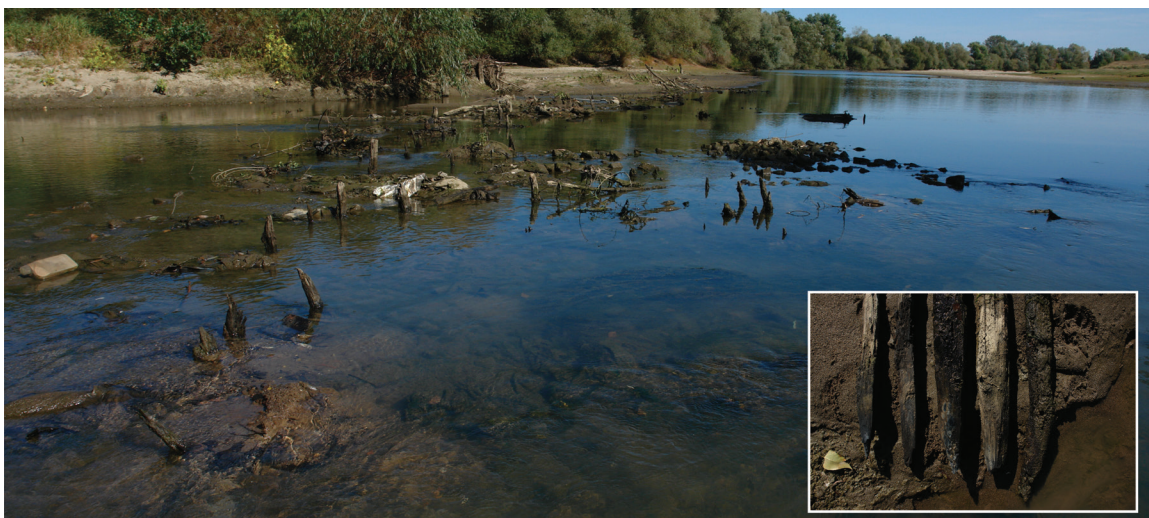
Fig. 38. Uliuc-Timiș 6. The alignment of poles forming the dam, view from the south (October 2019) and detail with the working of poles at the top (frame).
